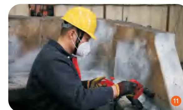
无损探伤 Non-destructive testing
