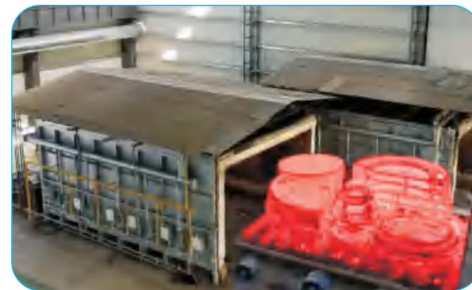
热处理窑2台 Two heat treatment kilns
