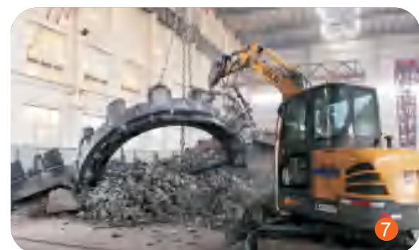
铸件清理 Casting Cleaning
